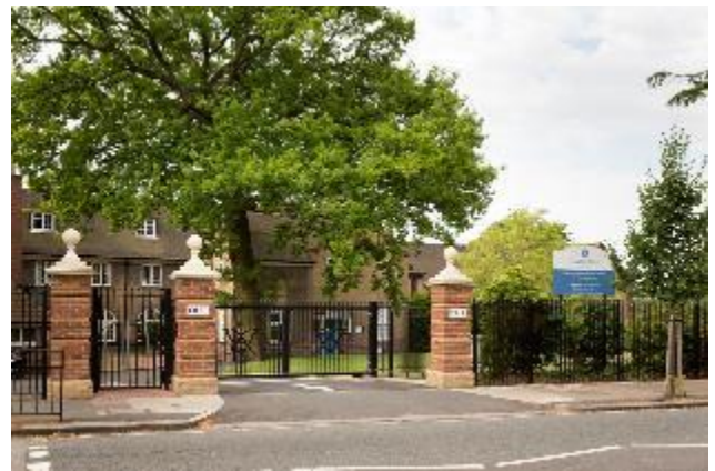
4. Secure entrance gates
