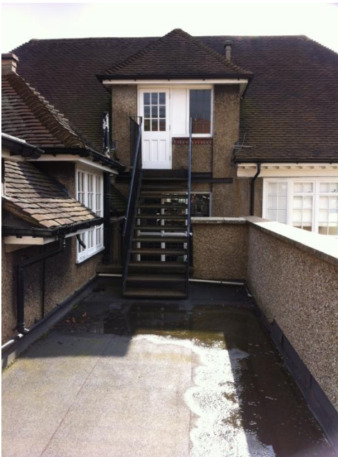
Wet weather matting has been added to improve area.
